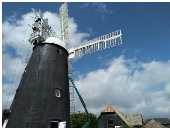
The Mill shutters were replaced in July
